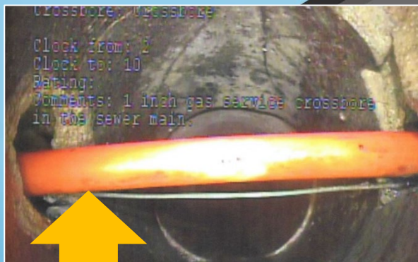
ACTUAL CAMERA FOOTAGE OF A CROSS-BORE
