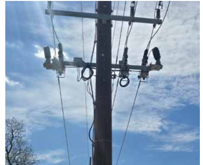
Distribution Automation controlled Viper Recloser.
