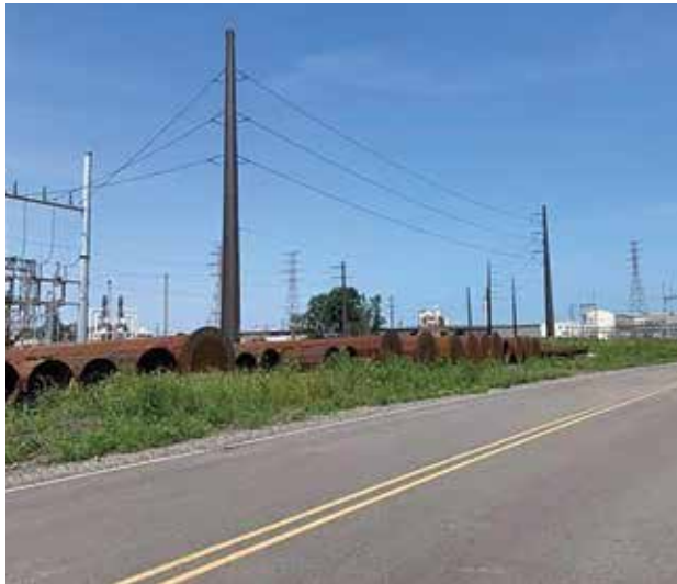
Steel mono-poles awaiting installation outside of Marktown Substation in Lake County, Indiana.
